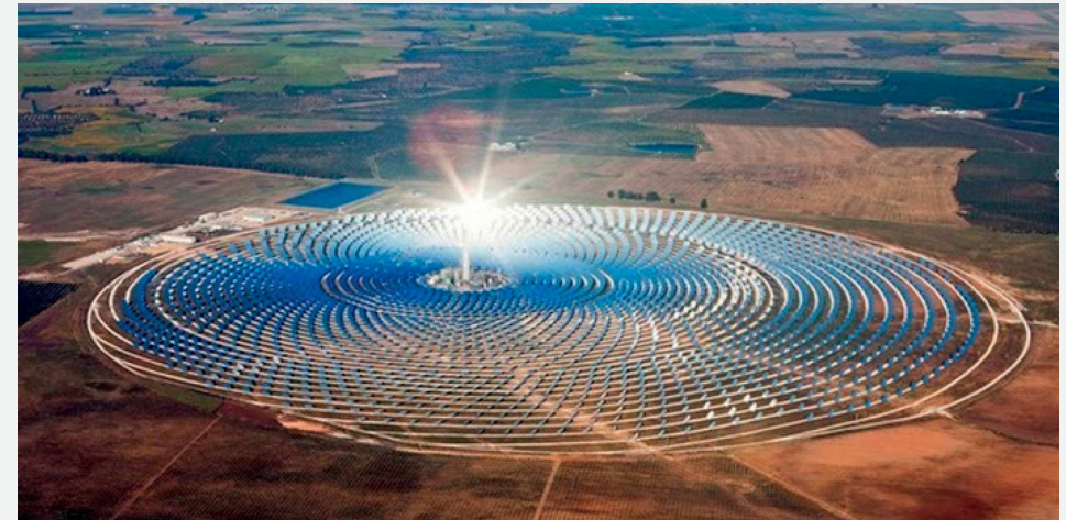
The Noor solar power plant in Ouarzazate
